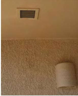
Your home may be equipped with a **washable** air filter that is usually located in the fresh air vent on your front porch (pictured here). But it can also be located behind the replaceable filter in your hallway. You will need a Phillips head screw driver to remove the two screws holding the grill in place and then remove the filter, vacuum it, wash it with water with a bit of vinegar (to kill bacteria), rinse thoroughly, put it back in place and screw the grill back in place.
