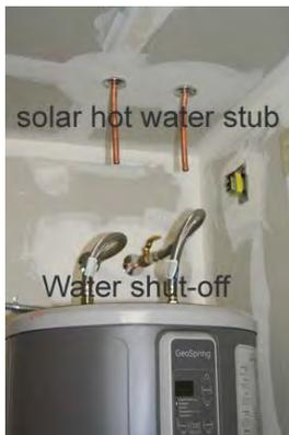
Your water heater is covered by a warranty from the manufacturer. Please read the operating instructions. In the event of a leak in your water heater, close the shut-off valve on the top of the water heater and turn off the circuit breaker located in the circuit breaker panel.
