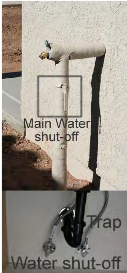
The main water shut-off is located below the front hose bibb. The valve shown in the picture is in the ON position and water can flow into the house, simply turn the handle to turn off the water. Our representative will identify the water shut-off during your walkthrough.
