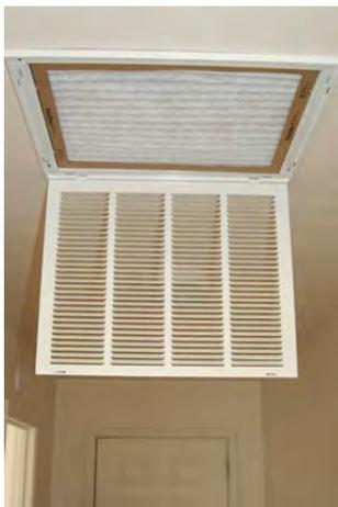
We recommend that the replaceable ***filters be changed every 30 days***. Your replaceable filter is usually located behind a large grill in your hallway ceiling, but this can vary from house to house. In areas with heavy dust more frequent changes may be in order. Fresh filters will significantly reduce operating costs and will prolong the life of your system. 90 day filters are available (and they cost more than 30 day filters).
