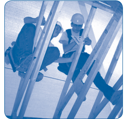
Stephen (right) works with a fellow student to secure the roof trusses.
